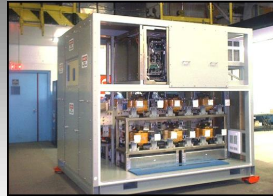
Navy Power Interface System With Electromechanical Assemblies
